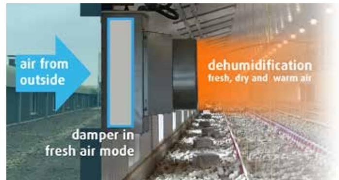
When the dampers in the unit are closed, the unit serves as a traditional heater, recirculating room air over the heater and distributing it evenly throughout the building.
