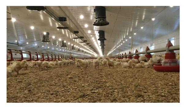
The patented **Corona** Inlet fan provides precise mixing of incoming air with warm room air, thereby maintaining a perfect in-house climate.
