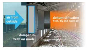
When dampers are open the unit serves as a heat exchanger and provides superior humidity control and ample supplies of preheated fresh air. The air entering the building is warm and will not cause draft or condensation. The air leaving the unit is extremely dry and will absorb moisture quickly and efficiently.
