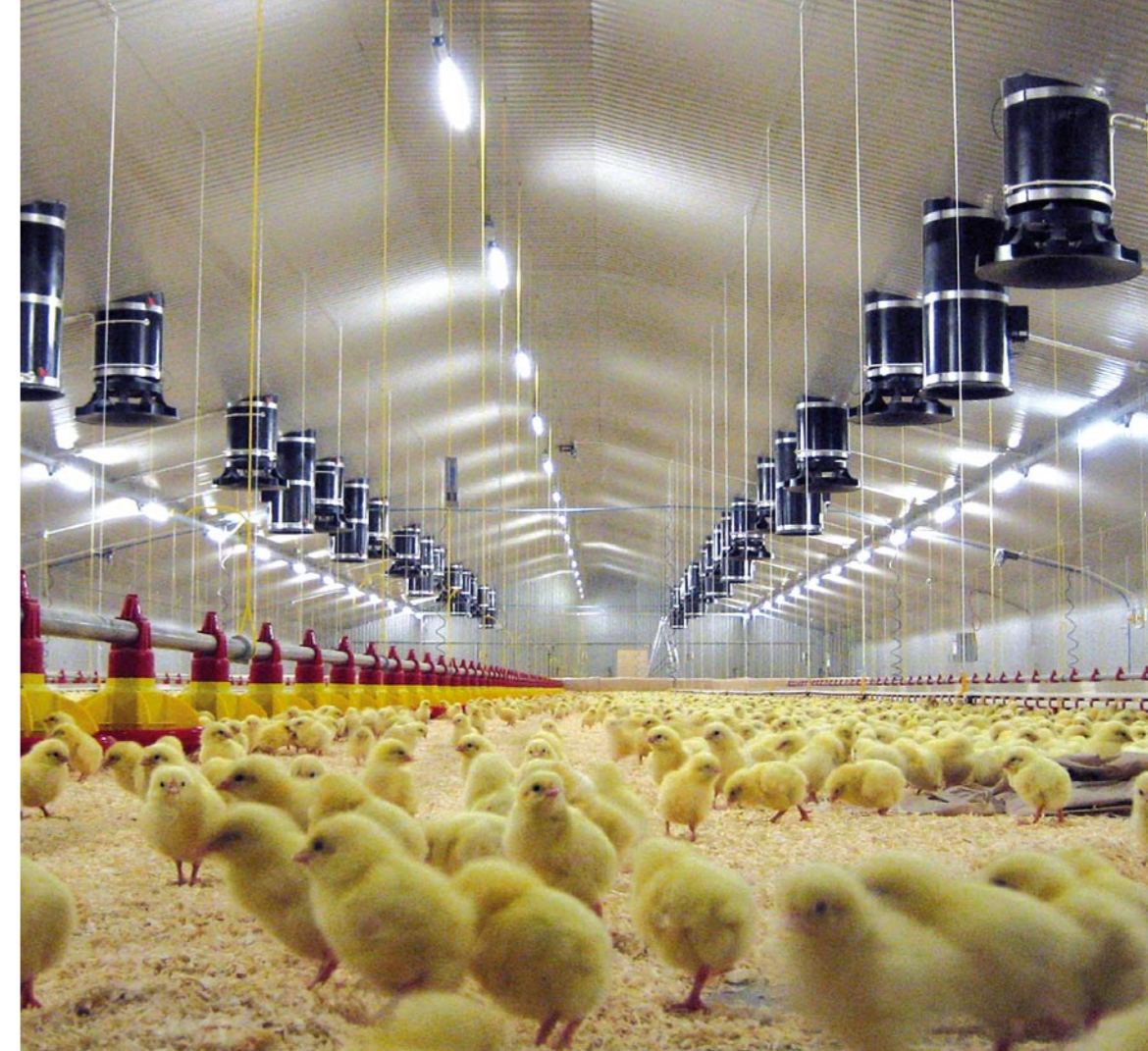
New chicks are benefiting from the improved litter quality seen with the Danish ventilation system.
